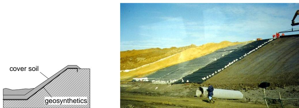
**Figure 38.** Geosynthetic layers in slopes of waste disposal areas.
