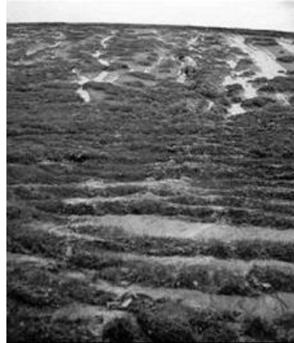
(b) Failure of cover soil (Gross et al. 2002)
